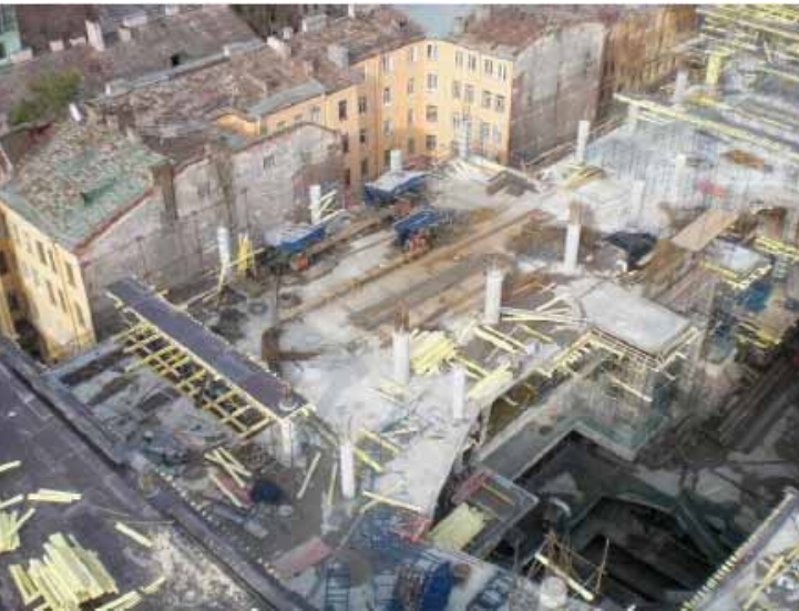
9 Oct 2009 Construction site from crane
